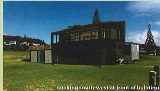
Looking south-west at front of building
