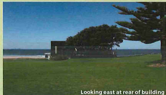
Looking east at rear of building
