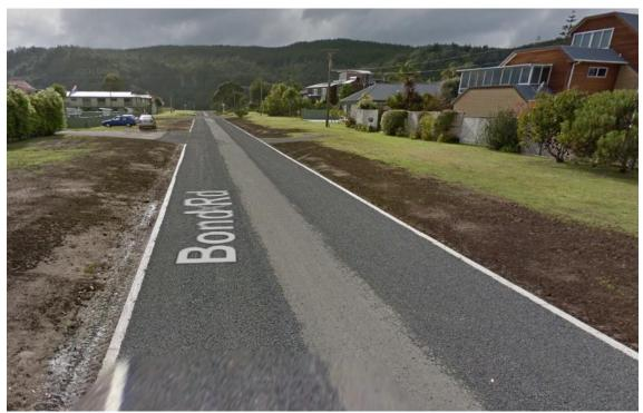
Nib kerb treatment is appropriate where the adjoing properties are higher than the road level and there is sufficient berm width to create a shallow swale for surface water runoff and soakage without significant earthworks.
